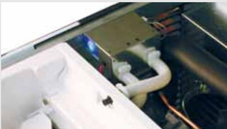
The LuminIce space-saving design fits inside the ice machine so existing exterior clearances are not impacted. In addition, power for the unit is supplied through the ice machine’s internal electrical supply so outlet space is conserved.
